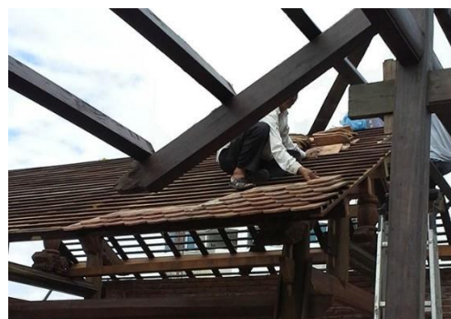
Fig. 10 Installation of roofing tile at a new residential construction
