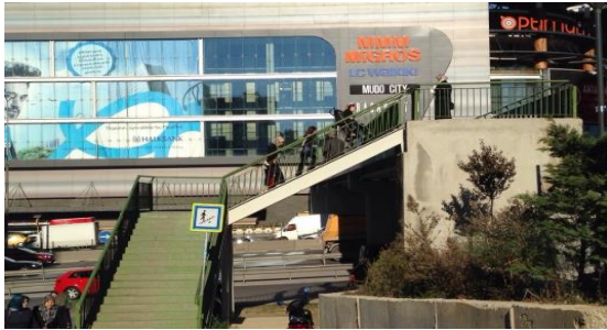
Figure 10: Stairs without any ramp, Ataşehir, İstanbul
