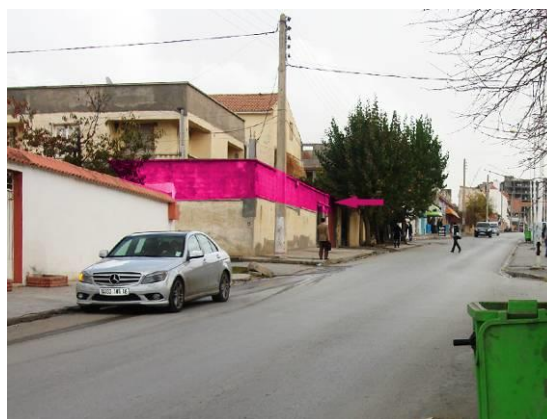
Photo 5: Extra height of fence (Screen) Source: The author (2014)
