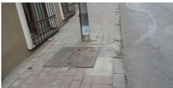
Figure 14: Barriers on pavement
