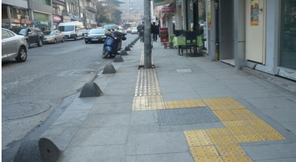
Figure 4: Electricity pylon on the yellow paving, Kadıköy, İstanbul
