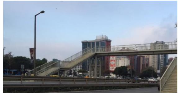
Figure 11: Stairs without any ramp, Ataşehir, İstanbul
