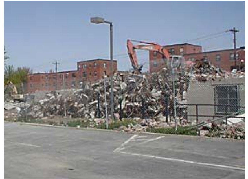
Public housing being demolished in Cincinnati
